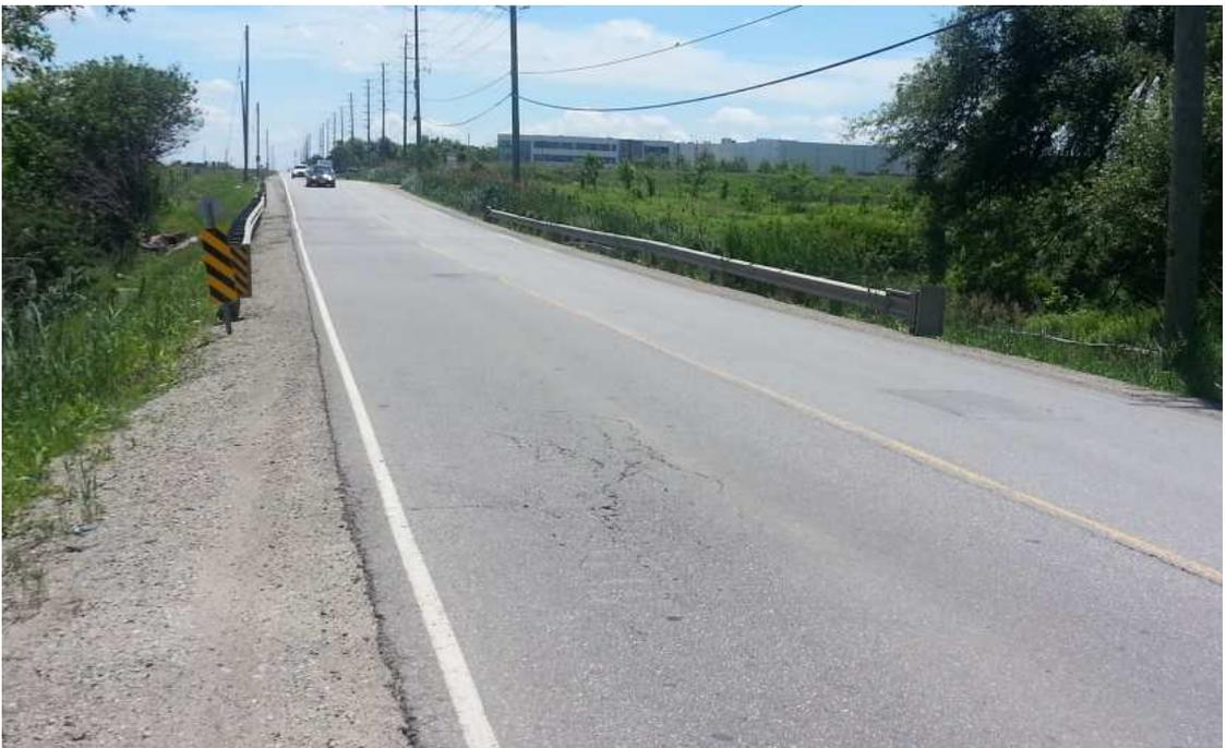
Photo 14: Slight to moderate map cracking and uneven surface of the road
