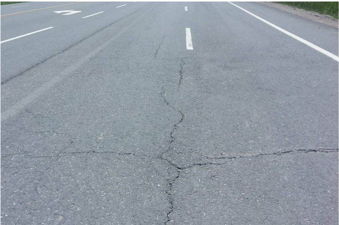
Photo 4: Slight to moderate transverse cracking
