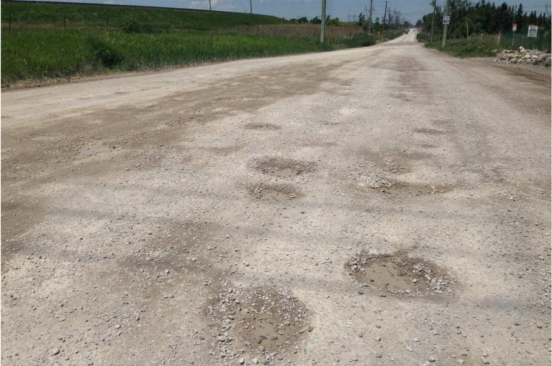
Photo 17: Potholes/waterpools and uneven surface of the gravelly road
