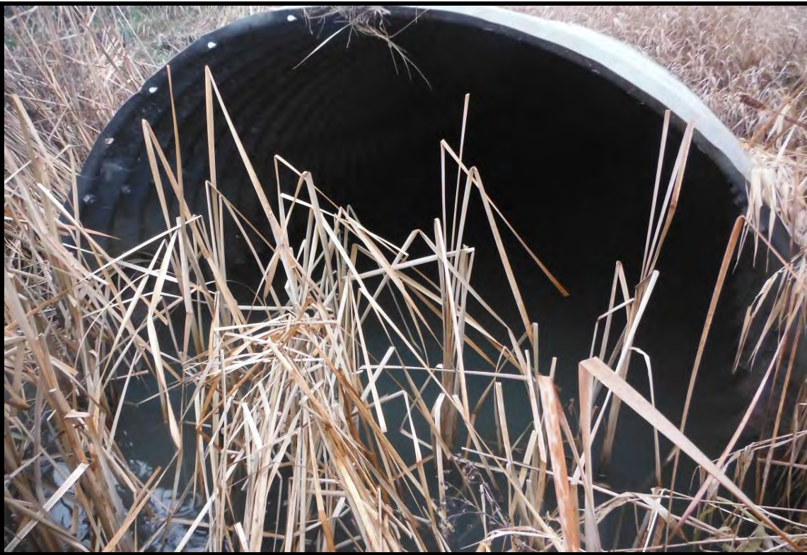
PHOTOGRAPH NO.: 11 - Culvert 6 FROM: Downstream end of culvert LOOKING: Upstream COMMENT:
