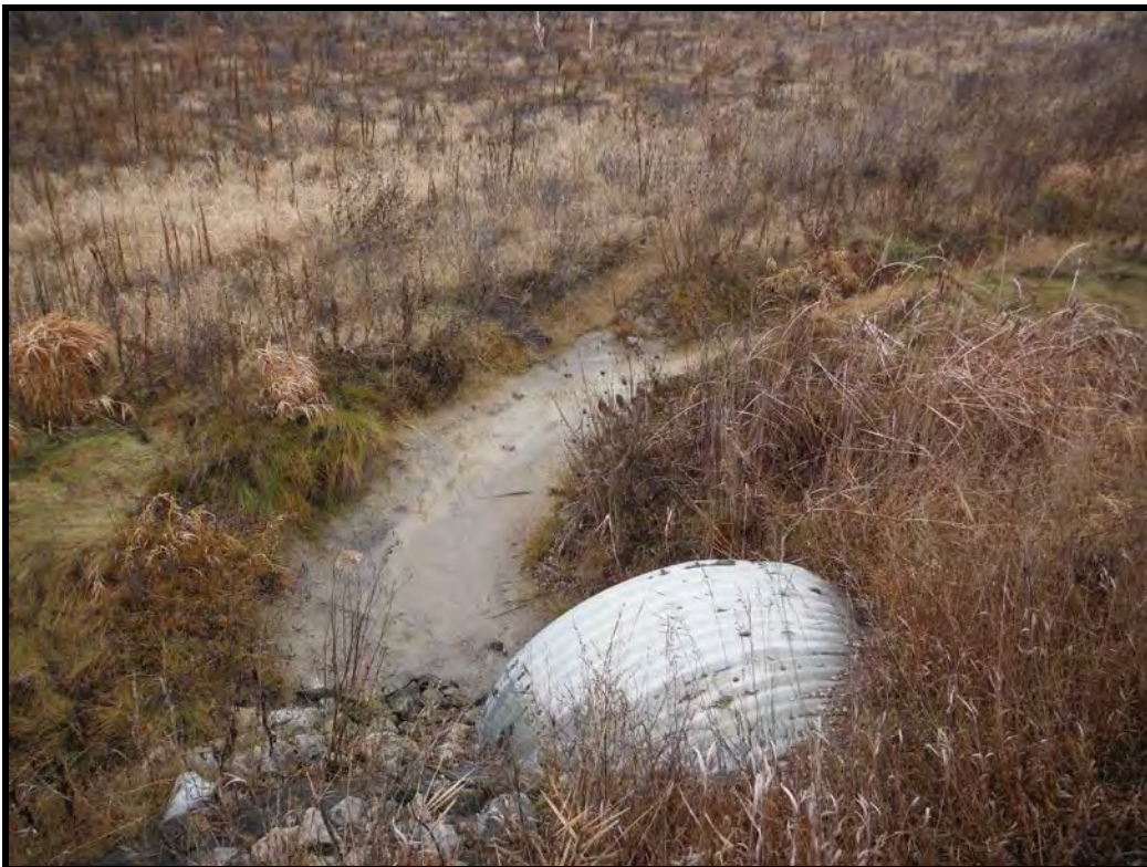
PHOTOGRAPH NO.: 2 - Culvert 4 FROM: Huntington Road LOOKING: Upstream COMMENT:
